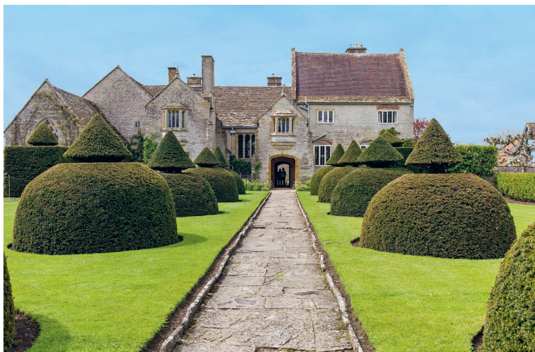
FIG. 8 Lytes Cary Manor in Somerset demonstrates the cellular principle on which early country houses were built. Rooms accreted around the great hall, the function of the different parts being plainly visible from the outside. The owners were a landed gentry family called Lyte with connections to the law. © Alamy
